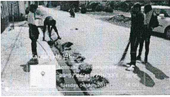
2021 - Drainage cleaning by the students
