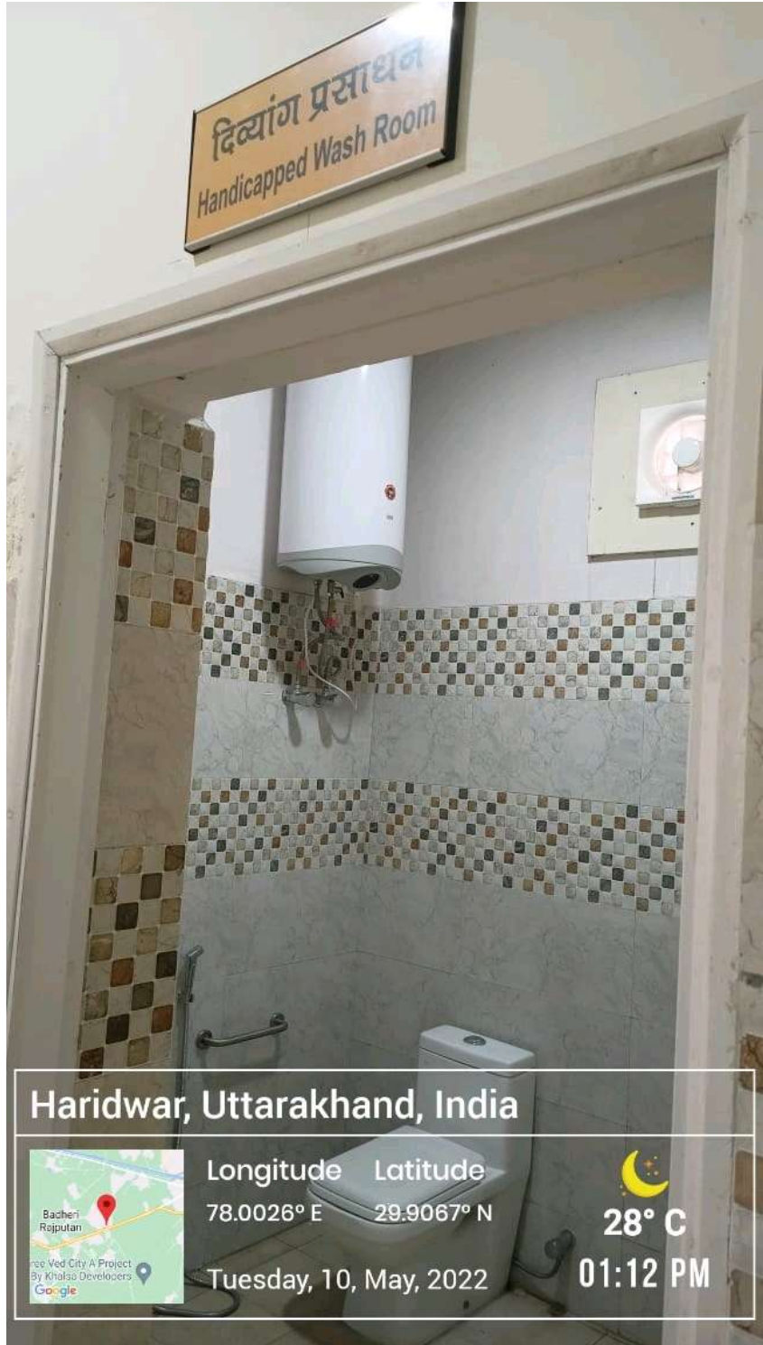
Divyang Washroom in University Hostel
