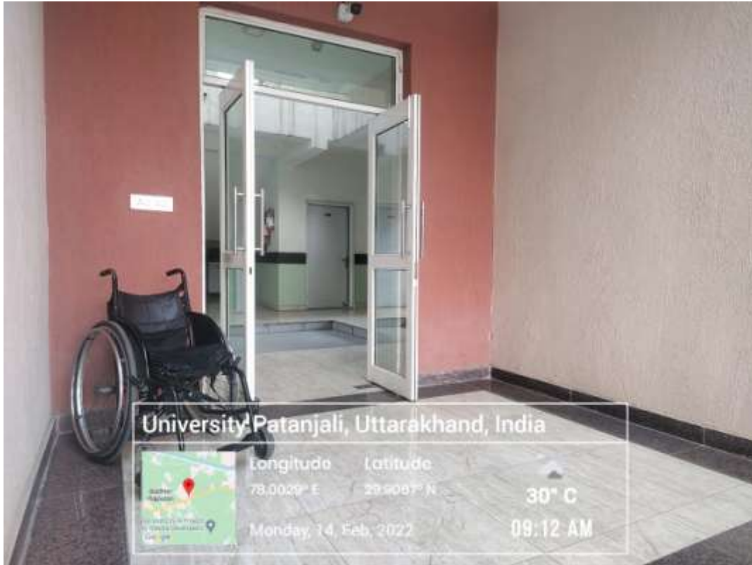
Wheel chair facility for divyangjan
