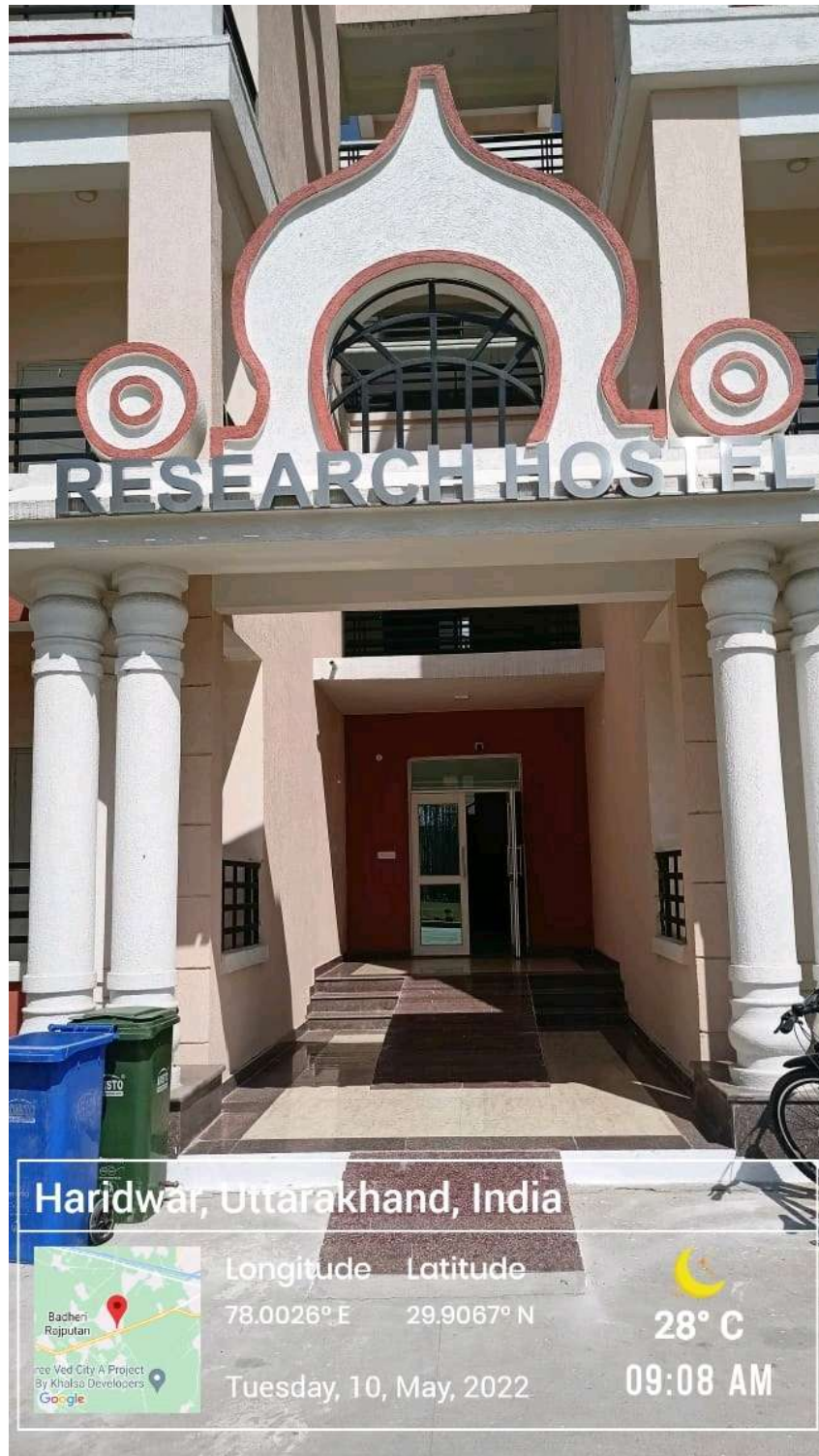
RAMP AT THE FRONT OF RESEARCH HOSTEL FOR DIVYANG SCHOLARS
